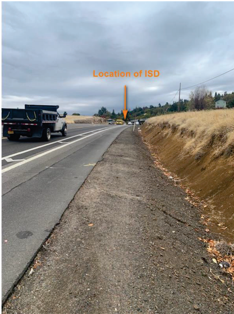
ISD requirement location looking north from site access. ISD is met
