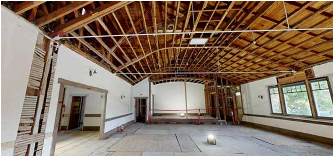
The interior of the Ashland Community Center after initial refurbishing work. City of Ashland photo
