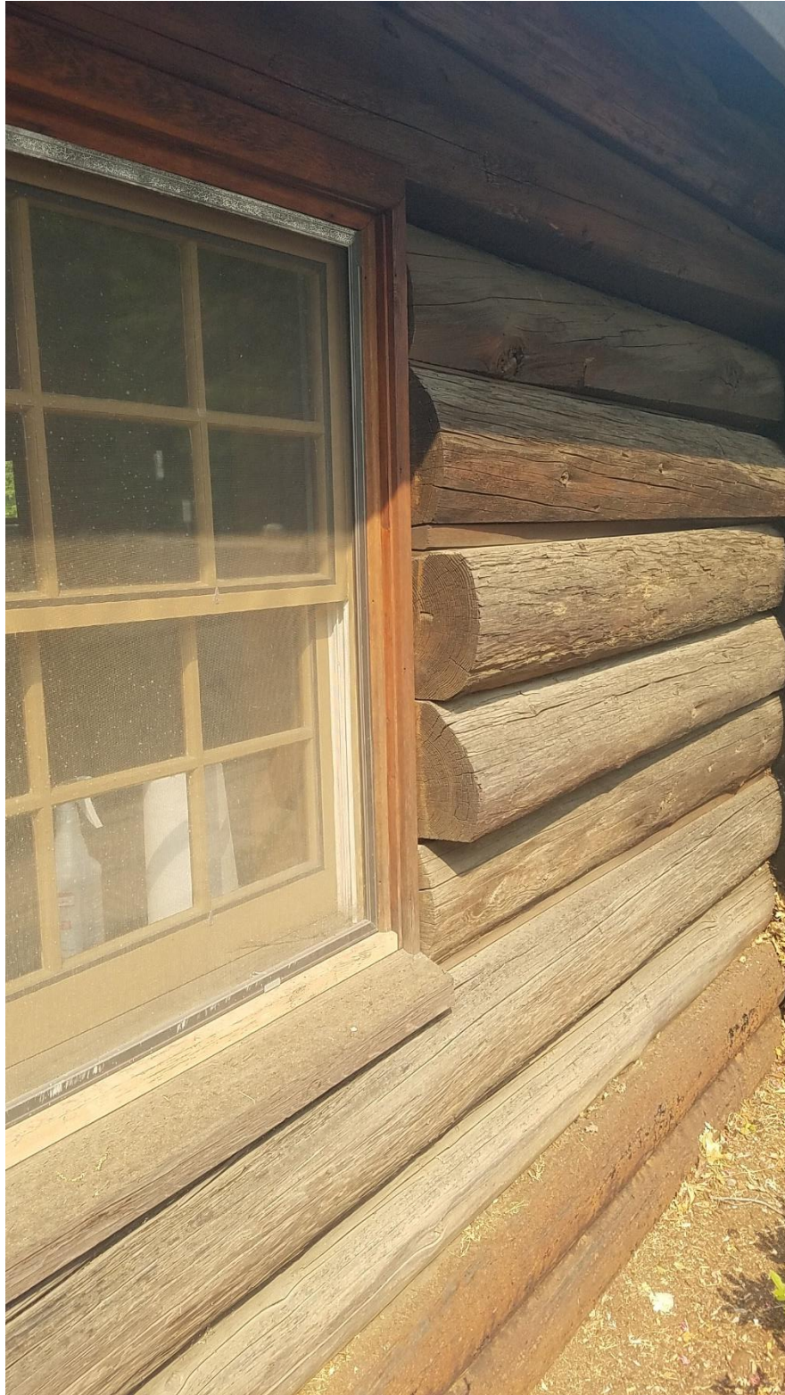
Figure 9. Pioneer Log Cabin, "Unpinned" Logs at SE Corner Window
