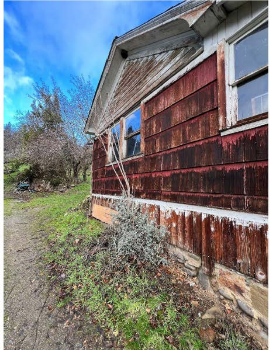
Figure 6: South Wall of house along the driveway
