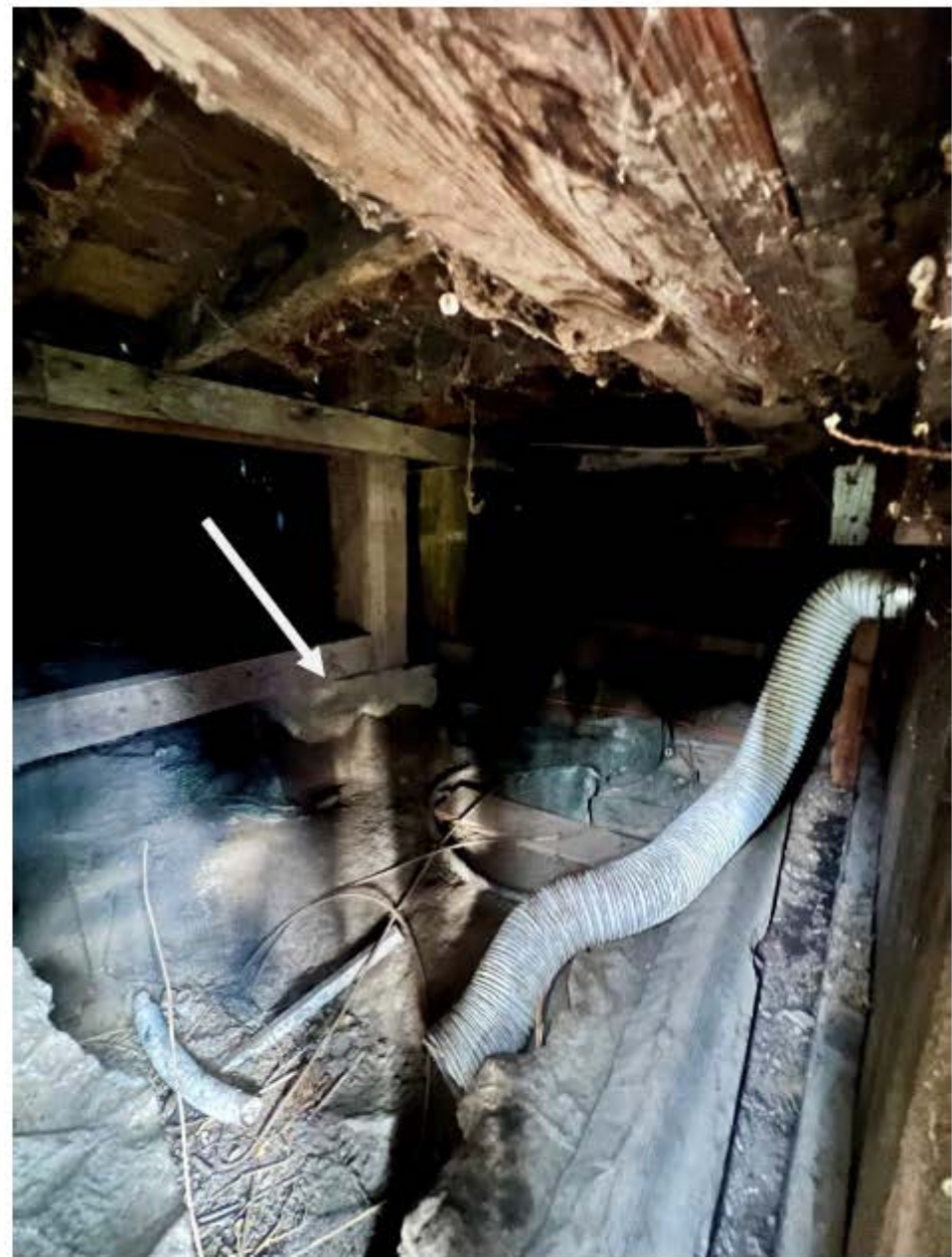
Figure 10: Rock stack supporting structure
