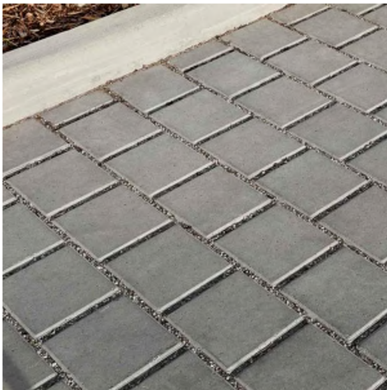
PERMEABLE PAVERS FOR PARKING STALLS
