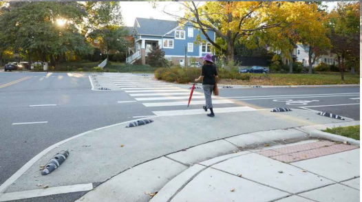
In the Near Term, Install Temporary Curb Extension
