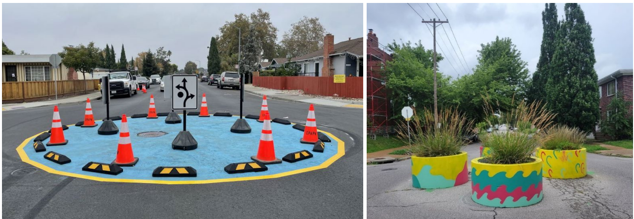
Figure 14. Quick-Build Traffic Circles
