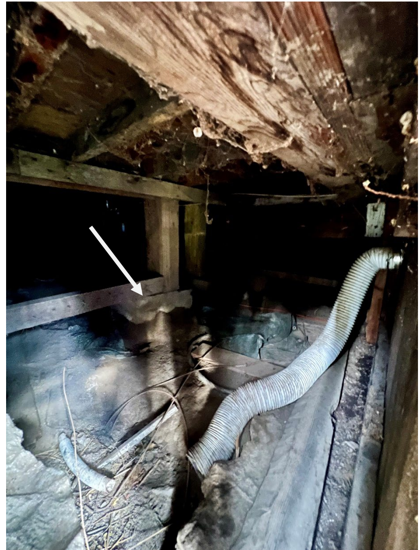
Figure 10: Rock stack supporting structure
