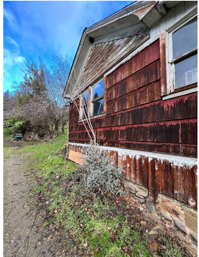
Figure 6: South Wall of house along the driveway
