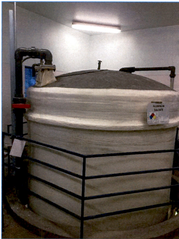
Photo 3-6 – Top of Alum Tank
