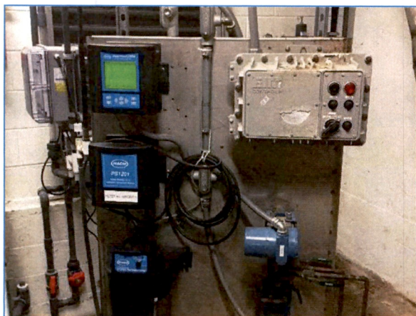
Photo 3-24 – Dual Media Filter #1 Turbidity Meter
