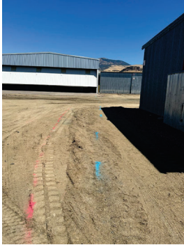
Pavement removal reveals unstable subgrade & base
