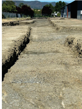
Unsuitable material is over-excavated, up to 18" deep
