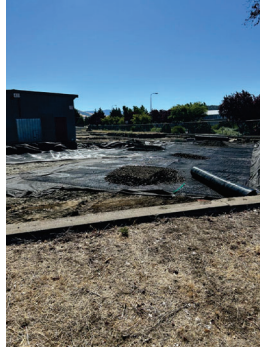
Geotextile, geogrid, and crushed rock are installed to stabilize subgrade & base
