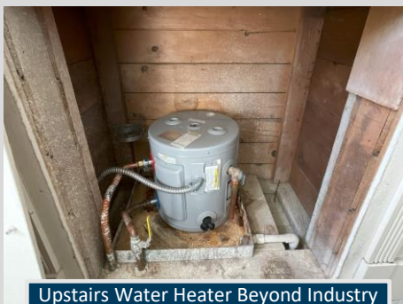
Upstairs Water Heater Beyond Industry Expected Life
