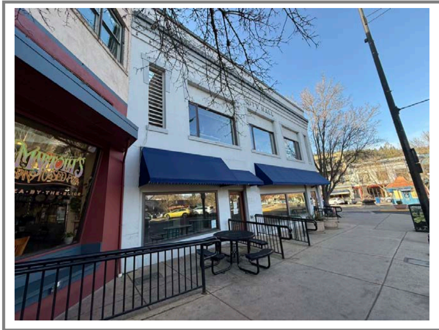
Additional front building elevation views
