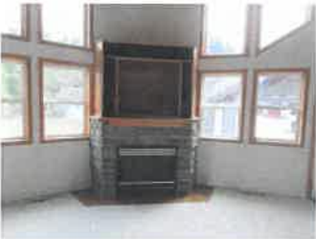
Living room gas fireplace
