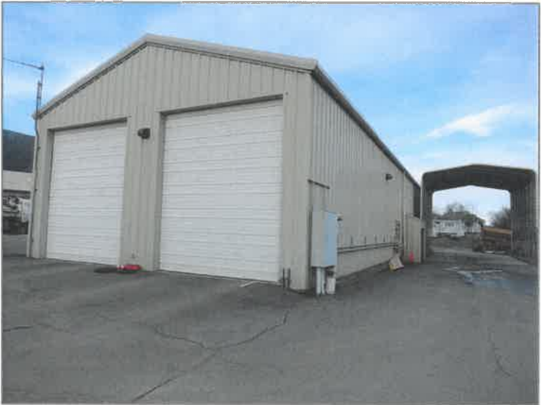
Northeasterly rear and side elevation of the larger building
