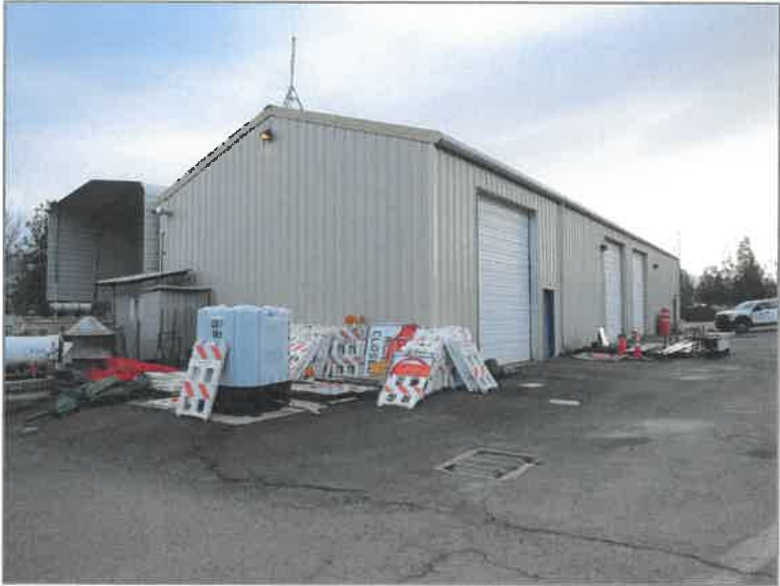
Southwesterly front and side elevation of the larger building
