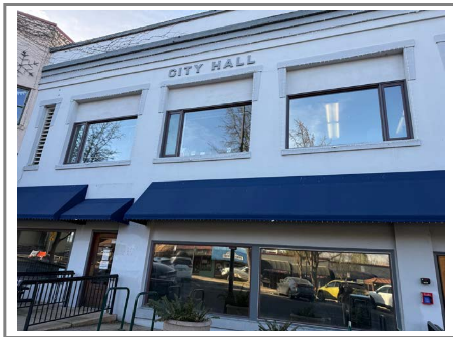
View of front building elevation from E. Main Street
