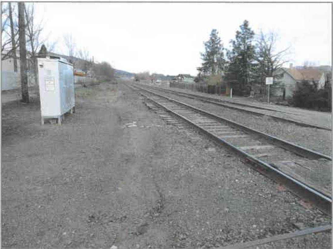
View of the railroad tracks on the north side of the subject, north of the bike path
