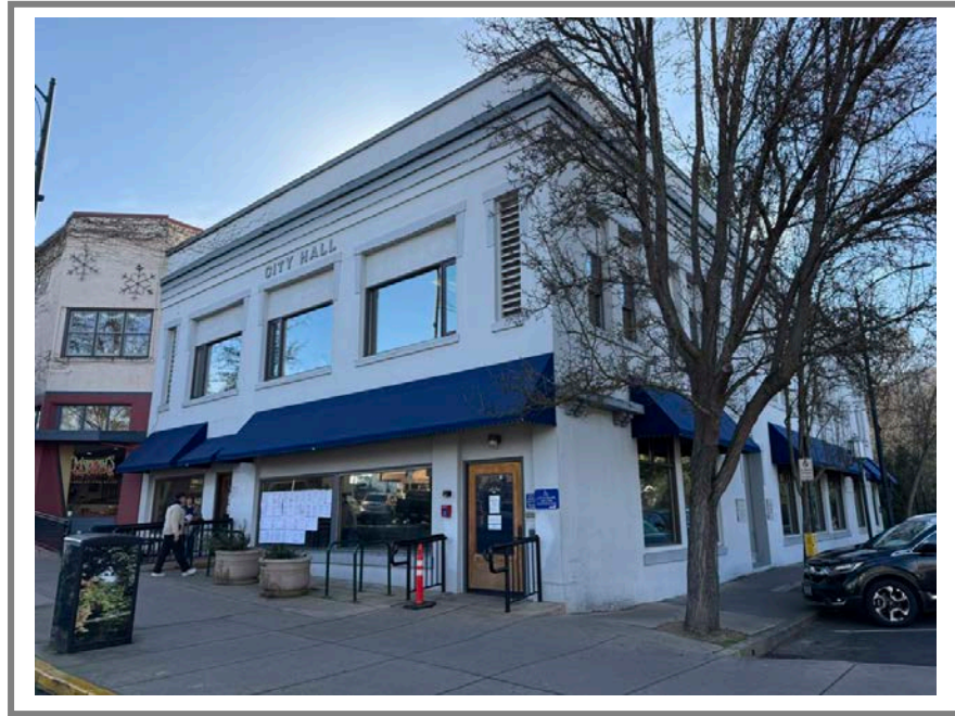
View of front and side (westerly) building elevations
