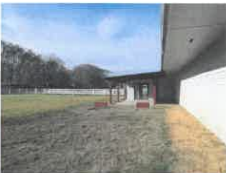
West elevation of gar, shp, off
