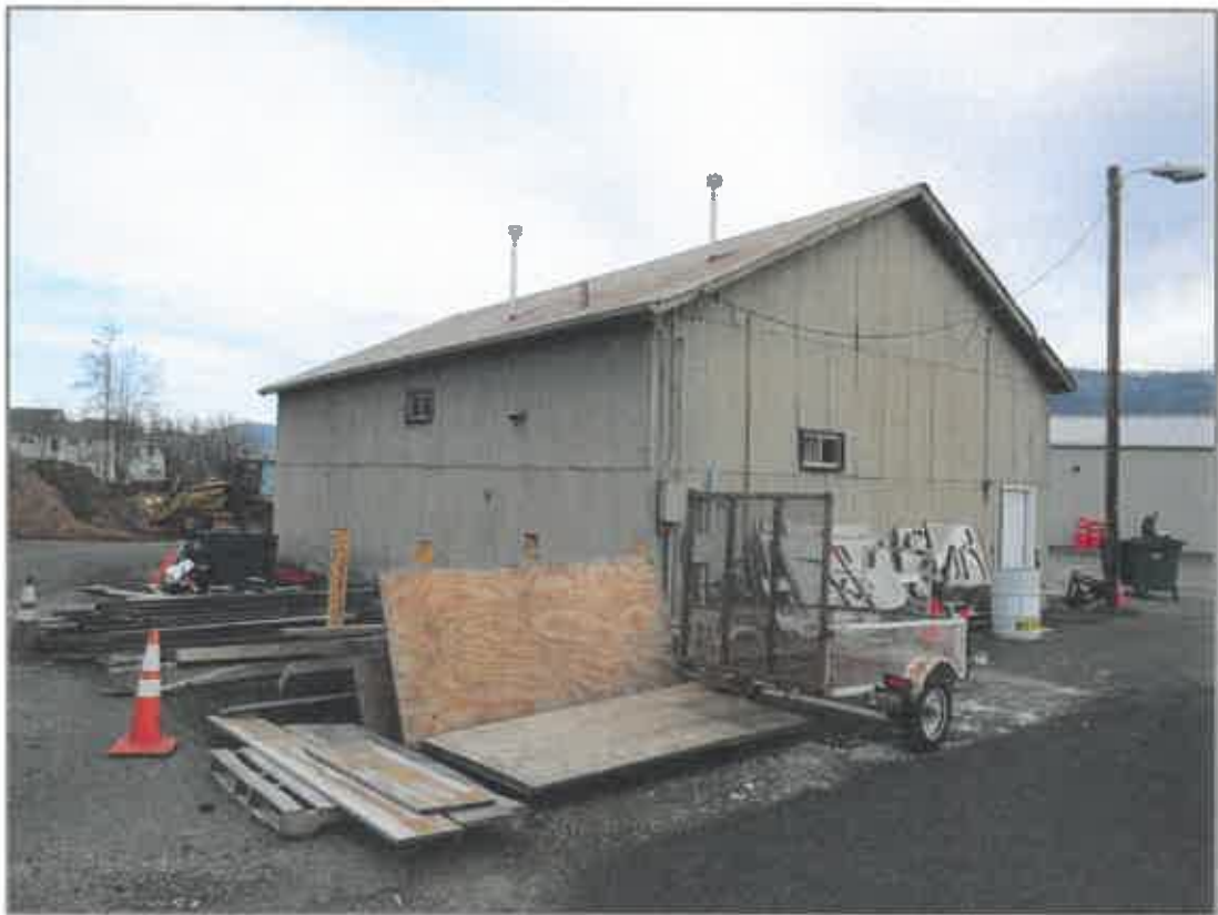
Southeasterly rear and side elevation of the smaller building
