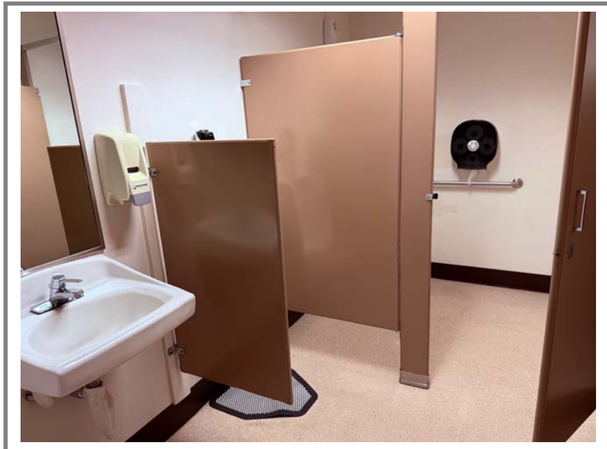
First floor men's restroom
