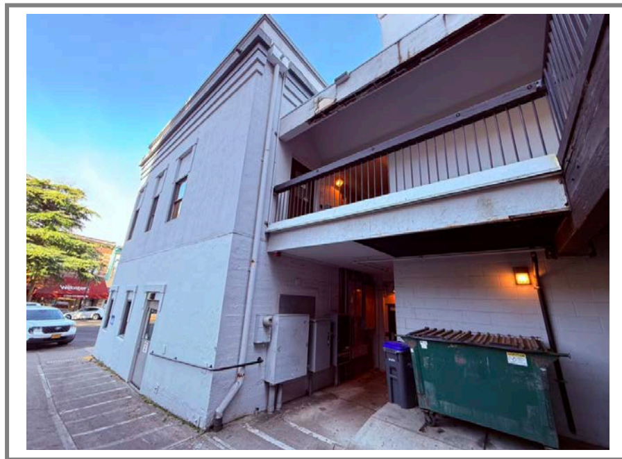
View of rear building elevation
