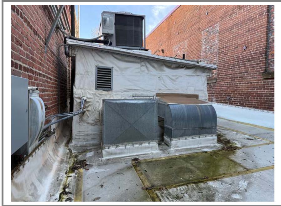
Views of roof area and mechanical equipment
