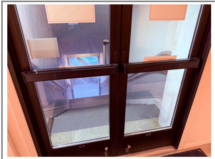
View of stairwell on west side of facility to exterior
