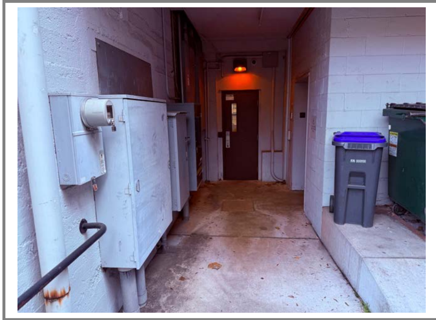
View of rear entry
