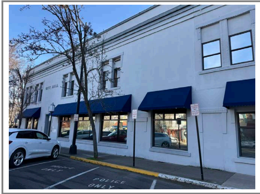
Additional side (westerly) building elevation from Plaza Loop
