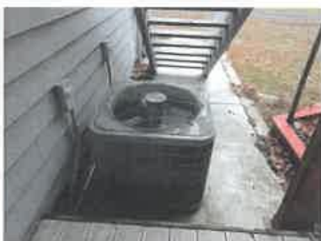
Cooled air compressor
