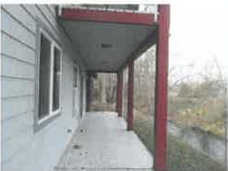
Creek view deck
