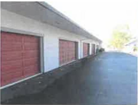
10 car garage, shop, office
