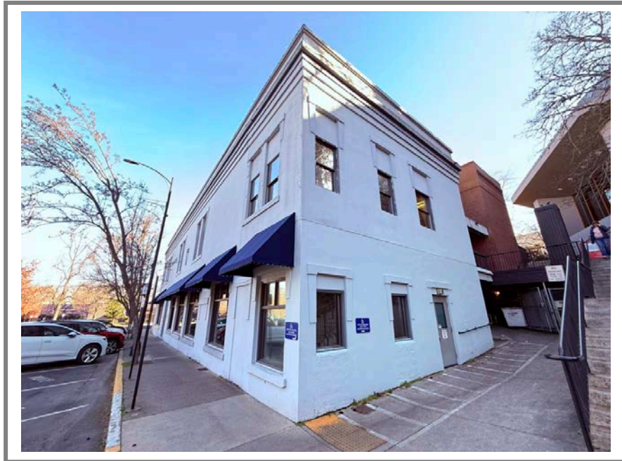
View of rear and side (westerly) building elevation
