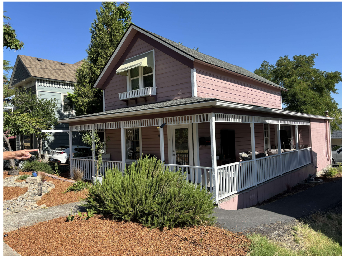
581 EAST MAIN STREET - STREET FACING EXISTING STRUCTURE
