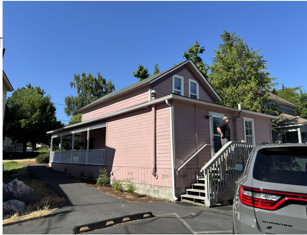
581 EAST MAIN STREET - ALLEY FACING EXISTING STRUCTURE
