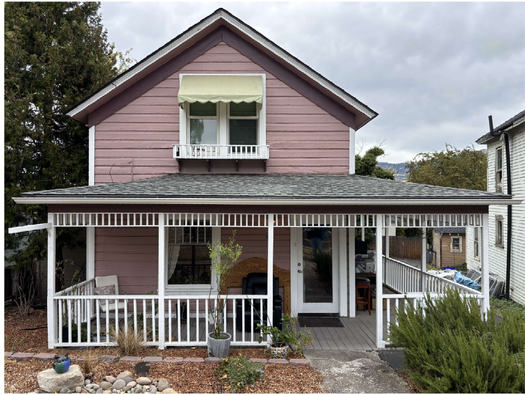
581 EAST MAIN STREET - STREET FACING EXISTING STRUCTURE
