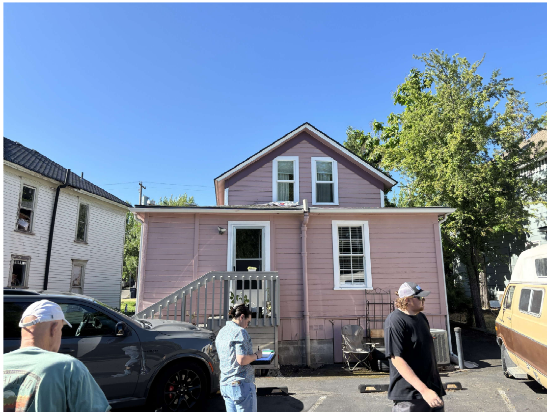
581 EAST MAIN STREET - ALLEY FACING EXISTING STRUCTURE
