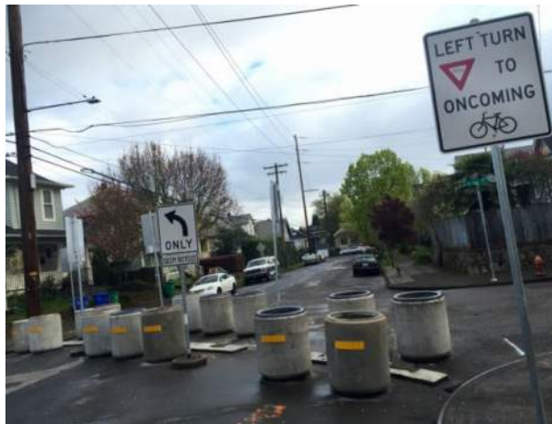
Diagonal Diverter with Concrete Barrels. Source: BikePortland
