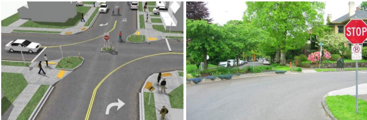
Figure 14. Traffic Diversion: Diagonal Diverters
