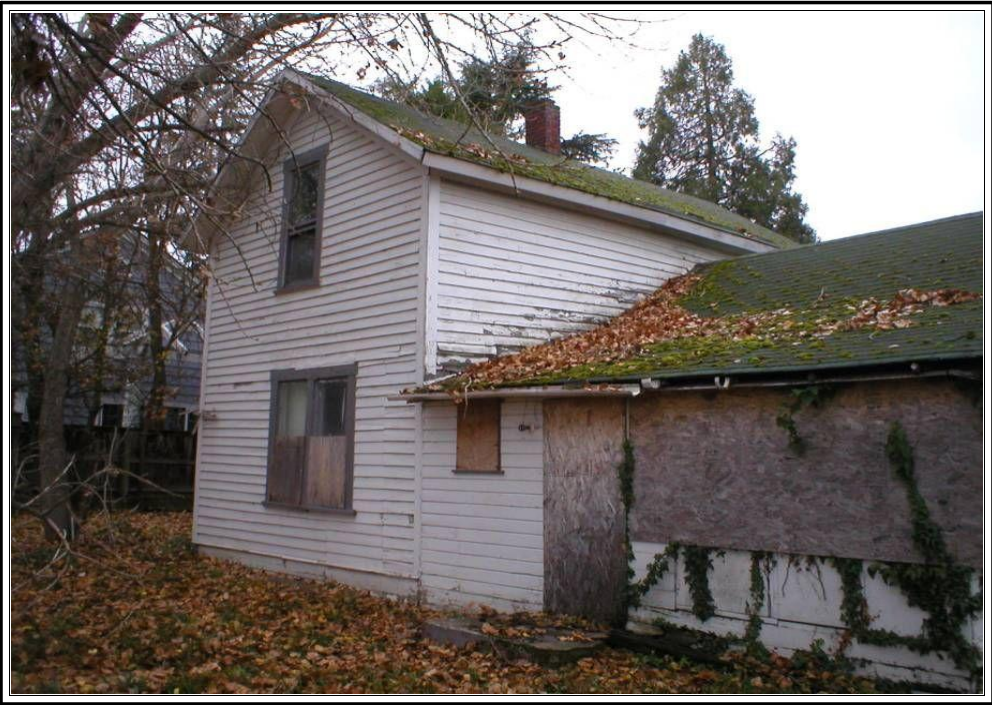
REAR OF SUBJECT PROPERTY
