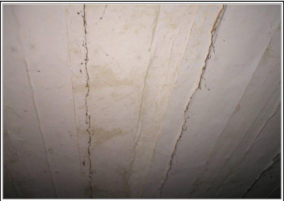
finished attic ceiling
