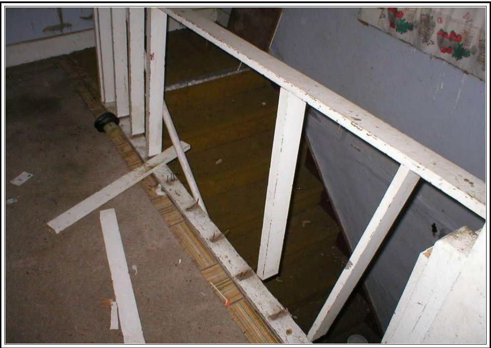
railing along stairs in 2nd level tandem bedroom
