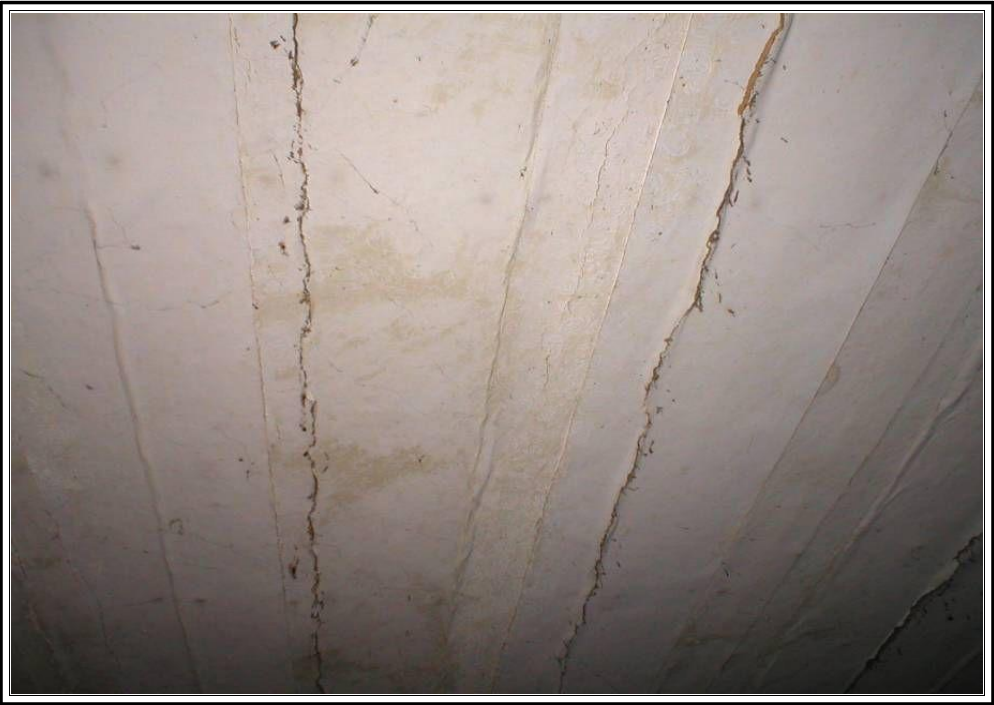
finished attic ceiling
