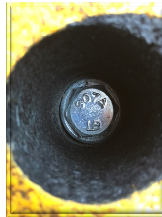
Properly seated lag bolt firmly on the washer.
