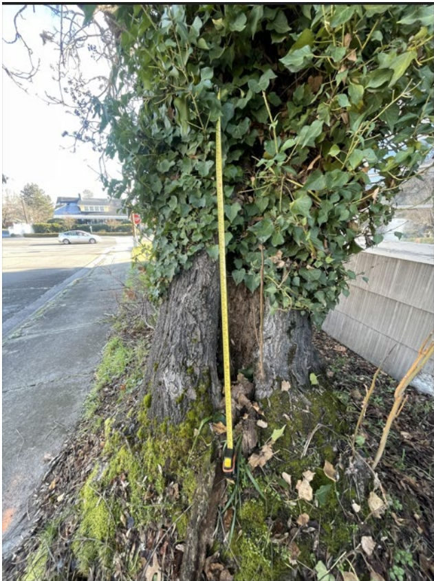
Staff Photo #1 – Cavity in the trunk of Tree of Heaven (Tape measure shows 47 inches)
