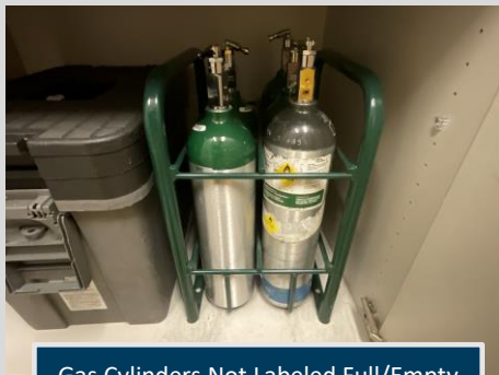
Gas Cylinders Not Labeled Full/Empty
