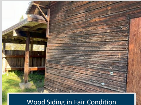
Wood Siding in Fair Condition
