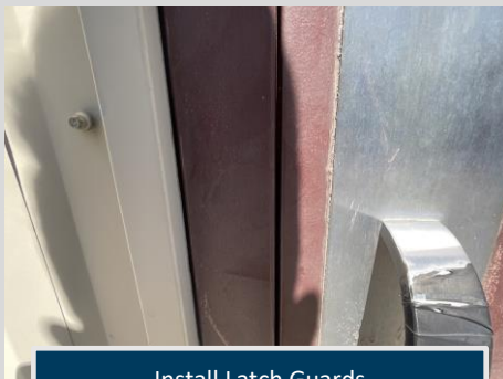
Install Latch Guards
