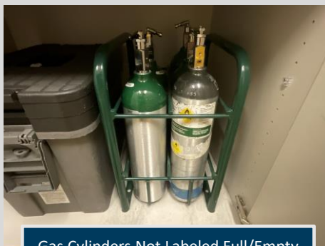
Gas Cylinders Not Labeled Full/Empty
