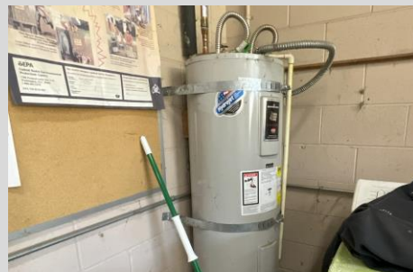
Softball Material and Equipment Storage Water Heater Exceeding Useful Life
