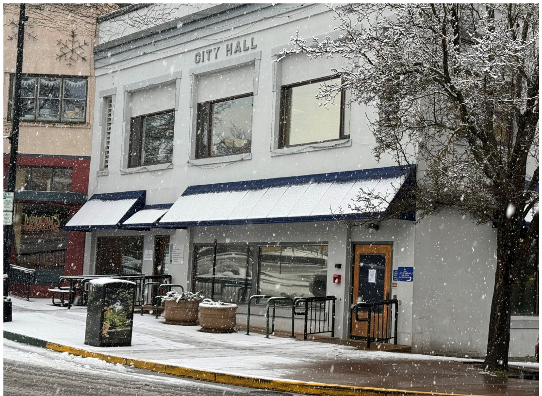
Right Ashland City Hall
