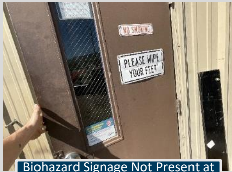
Biohazard Signage Not Present at Welding Shop
