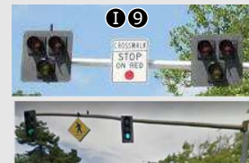
PED HYBRID BEACON (PHB) OR PEDESTRIAN SIGNAL
