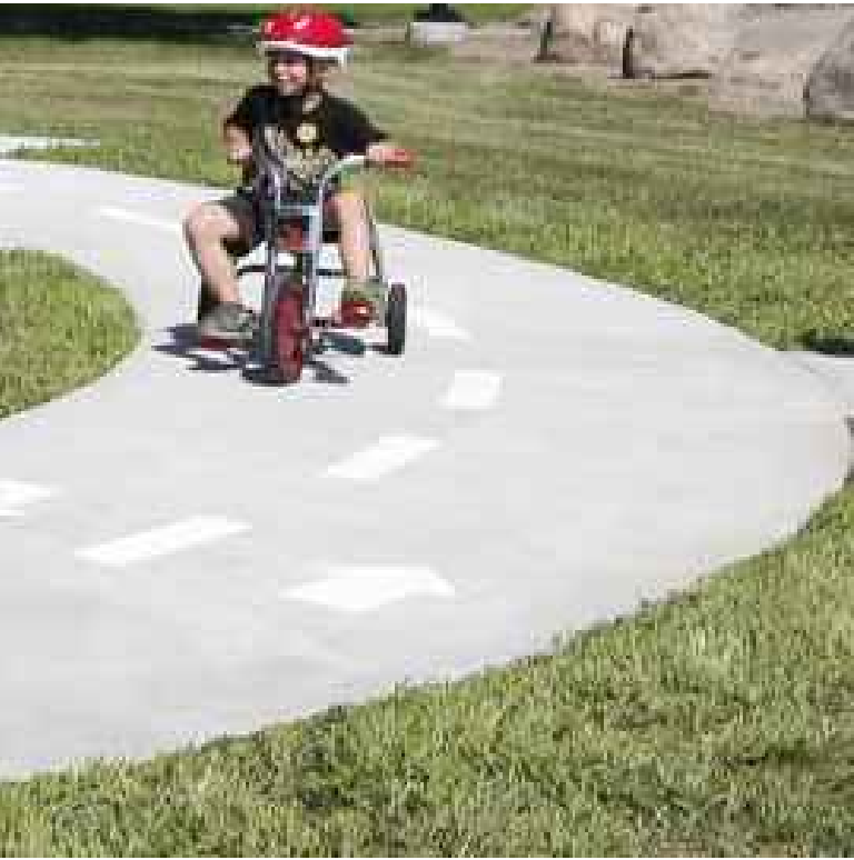
CONCRETE PAVING W/ PAINTED PLAY STRIPING
