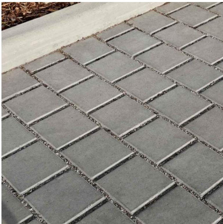
PERMEABLE PAVERS FOR PARKING STALLS
