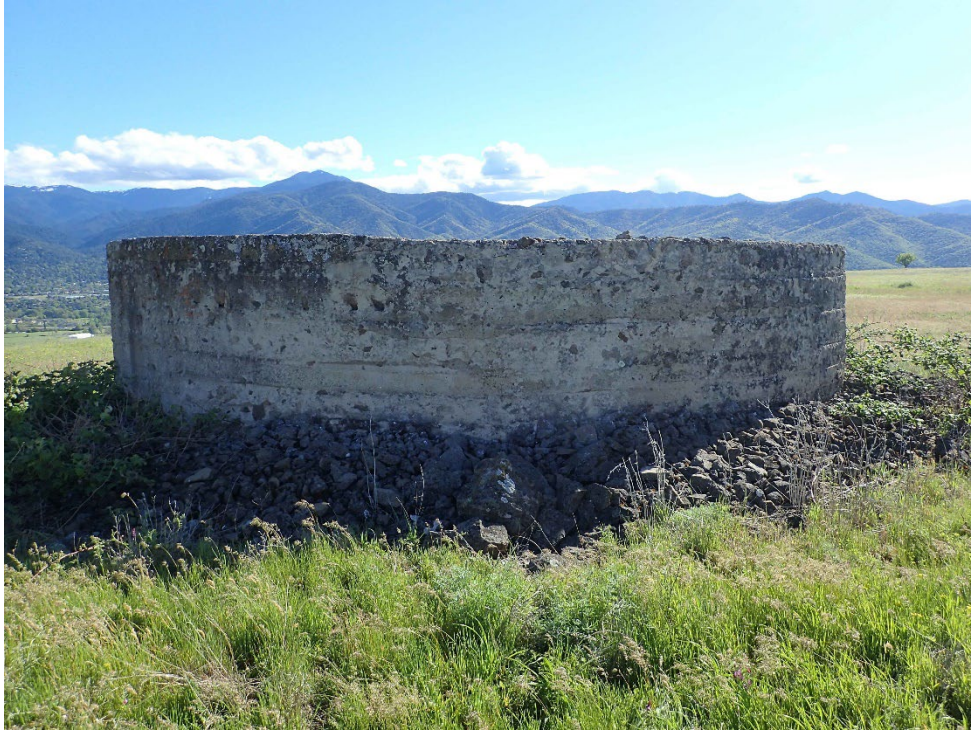
Cement “cistern” on broad ridgeline
