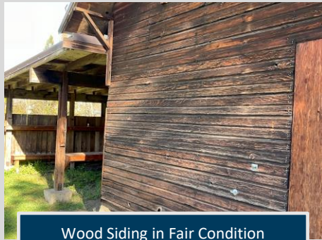
Wood Siding in Fair Condition
