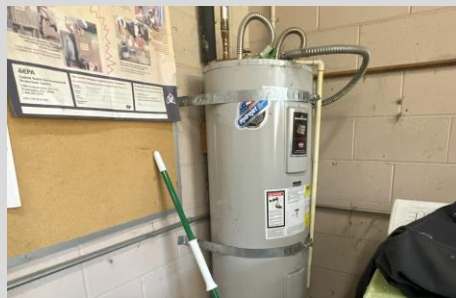
Softball Material and Equipment Storage Water Heater Exceeding Useful Life
