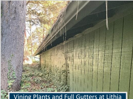
Vining Plants and Full Gutters at Lithia Park Material and Equipment Storage
