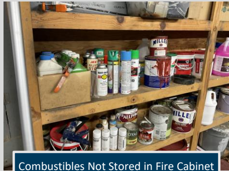
Combustibles Not Stored in Fire Cabinet
