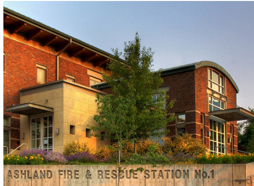
Right Ashland Fire & Rescue Station No. 1
