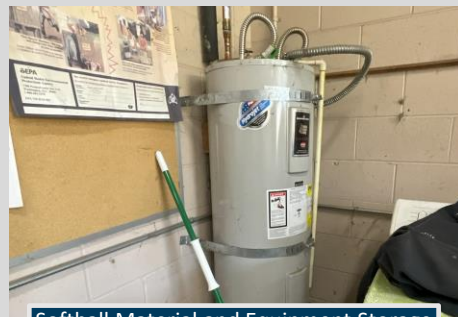
Softball Material and Equipment Storage Water Heater Exceeding Useful Life
