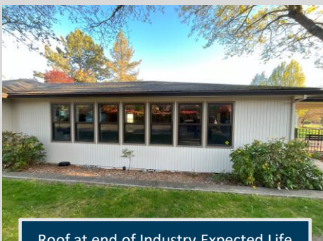
Roof at end of Industry Expected Life
