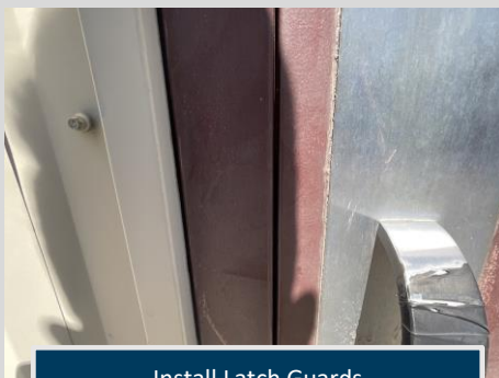
Install Latch Guards
