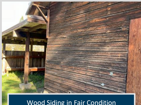
Wood Siding in Fair Condition
