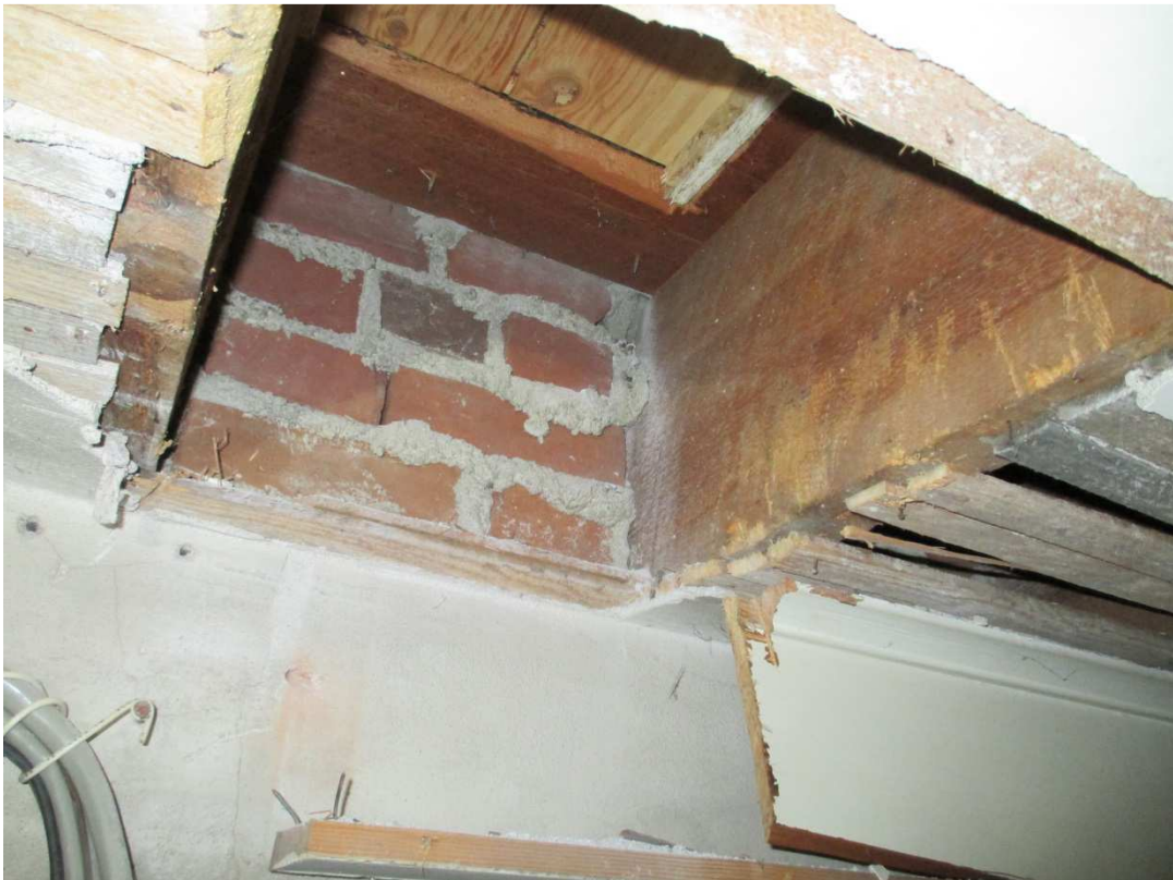
PHOTO 0242 – Upper floor connection at the east URM wall of the main building area
