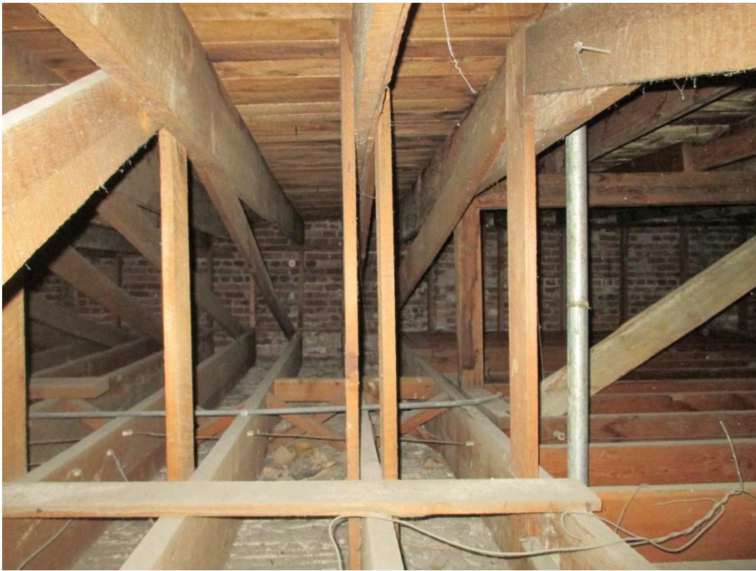
PHOTO 0256 – Main building area roof framing looking west
