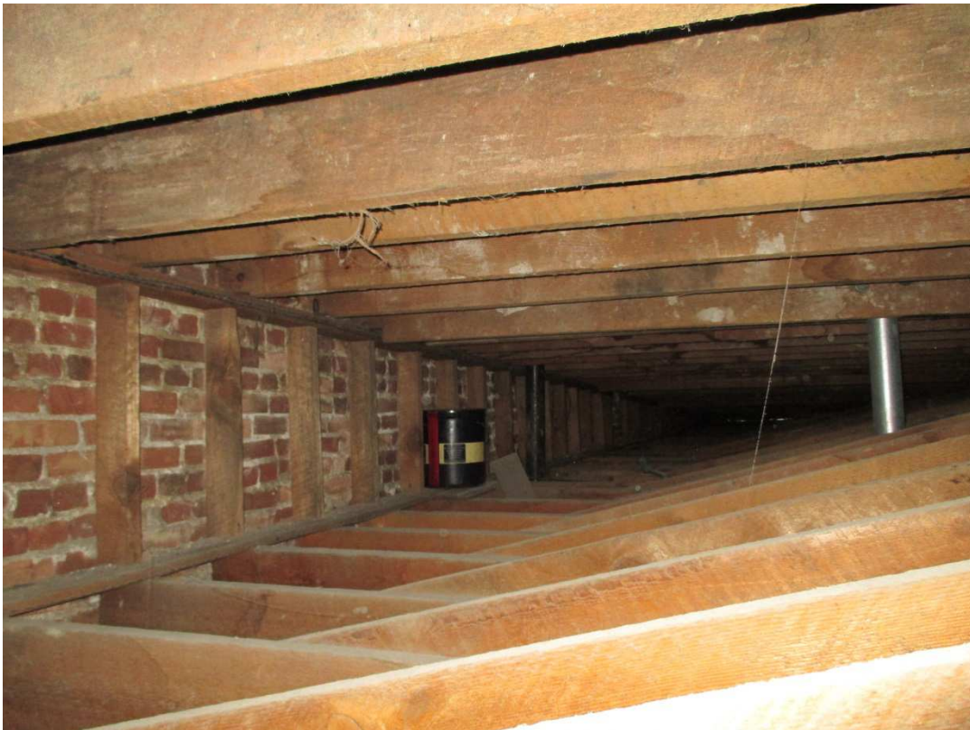
PHOTO 0264 – Main building area roof framing looking south
