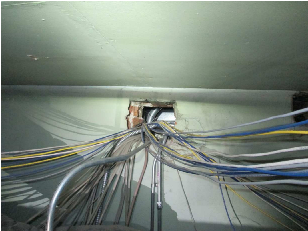
PHOTO 0235 – Access opening through the east URM wall in the main building area
