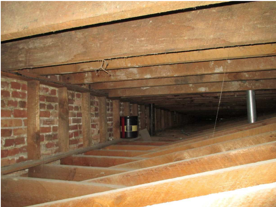
PHOTO 0264 – Main building area roof framing looking south
