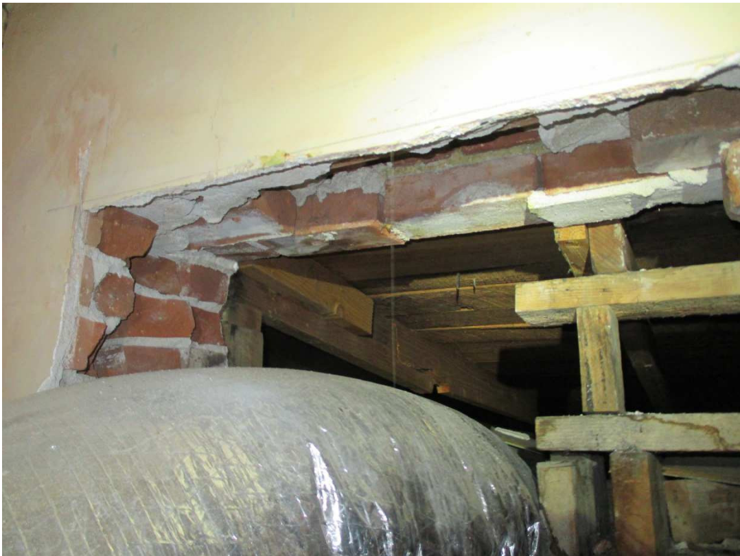
PHOTO 0261 – HVAC access in the upper floor ceiling cavity through the east wall
