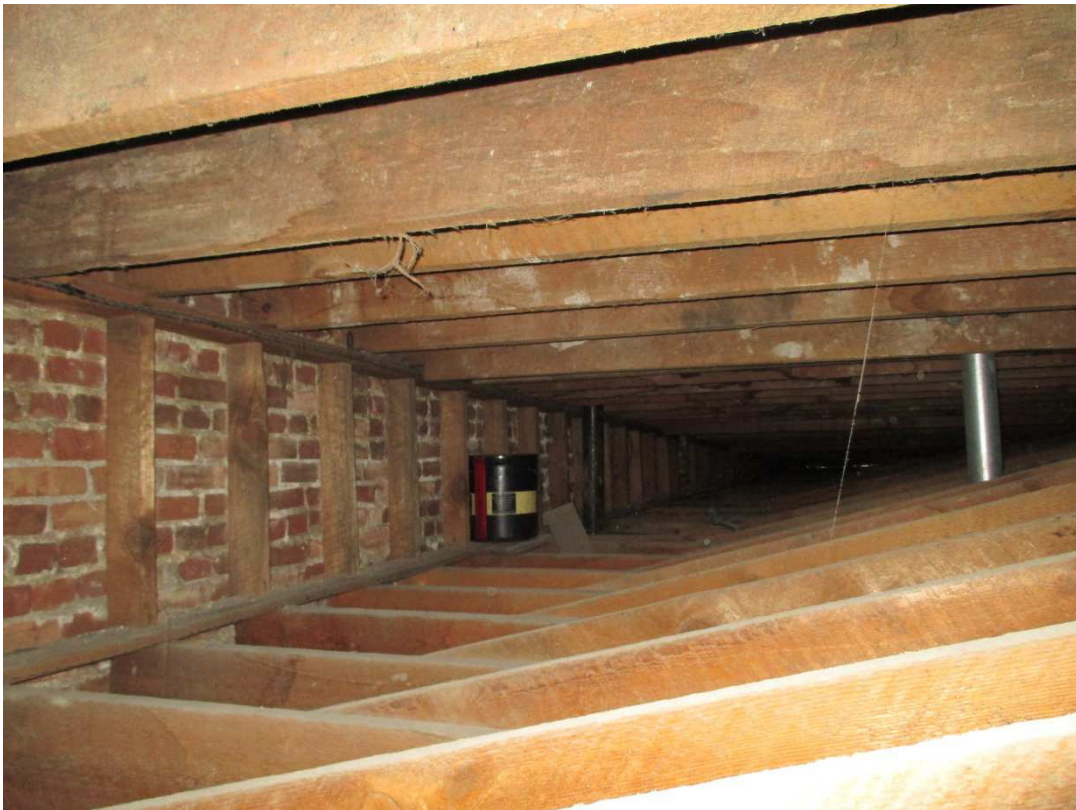
PHOTO 0264 – Main building area roof framing looking south
