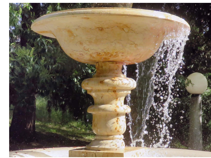
MARBLE FOUNTAIN UPPER PEDESTAL & BOWL REPLACE MARBLE UPPER PEDESTAL & BOWL W/ MARBLE TO MATCH EXISTING
