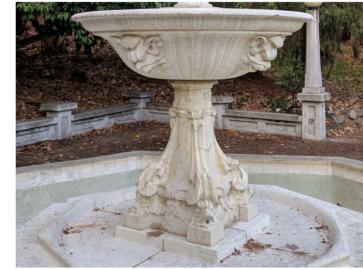
MARBLE FOUNTAIN LOWER PEDESTAL & BOWL 100 PERCENT OVERALL CLEANING OF EXISTING MARBLE TO BE REINSTALLED
