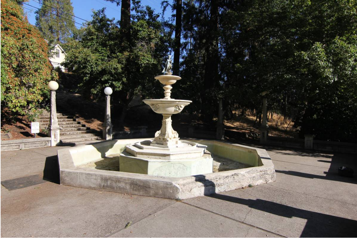
FIGURE 13. CURRENT IMAGE, Looking NW (note damage) G. Kramer Image, 2025
