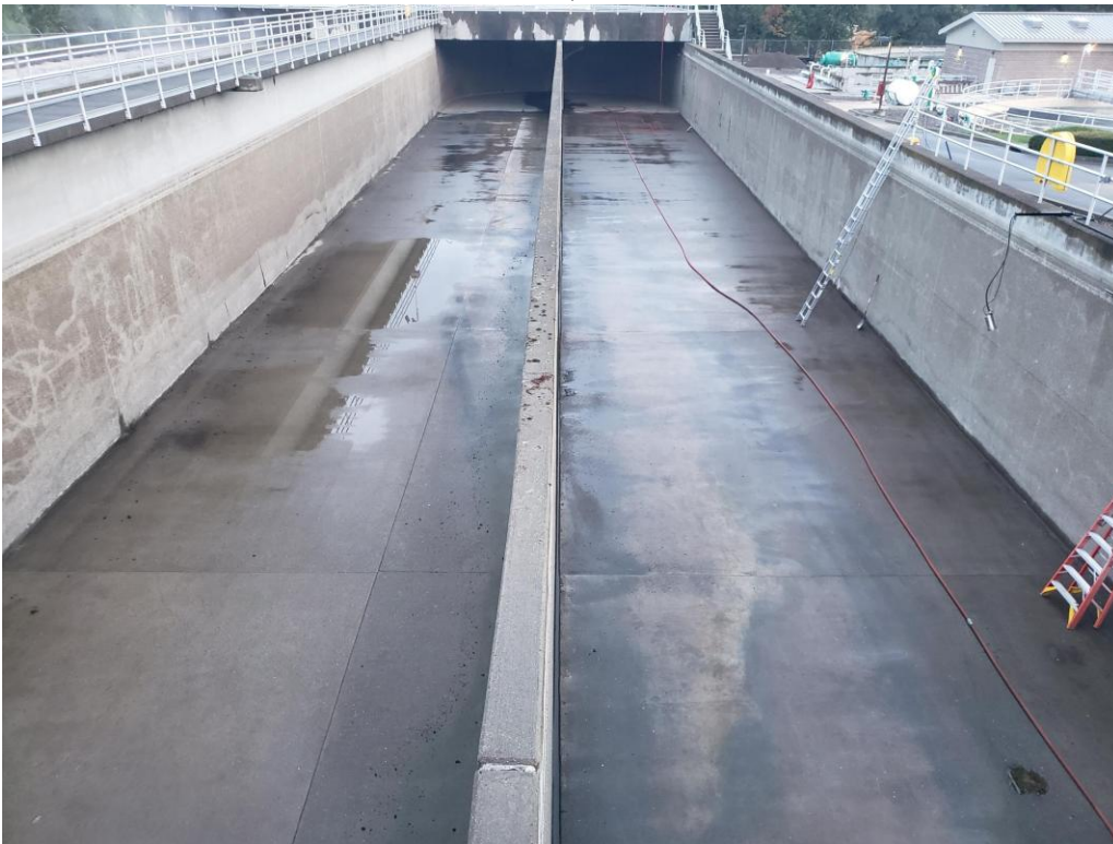
Cleaned out oxidation ditch at the City of Ashland Wastewater Treatment Plant
