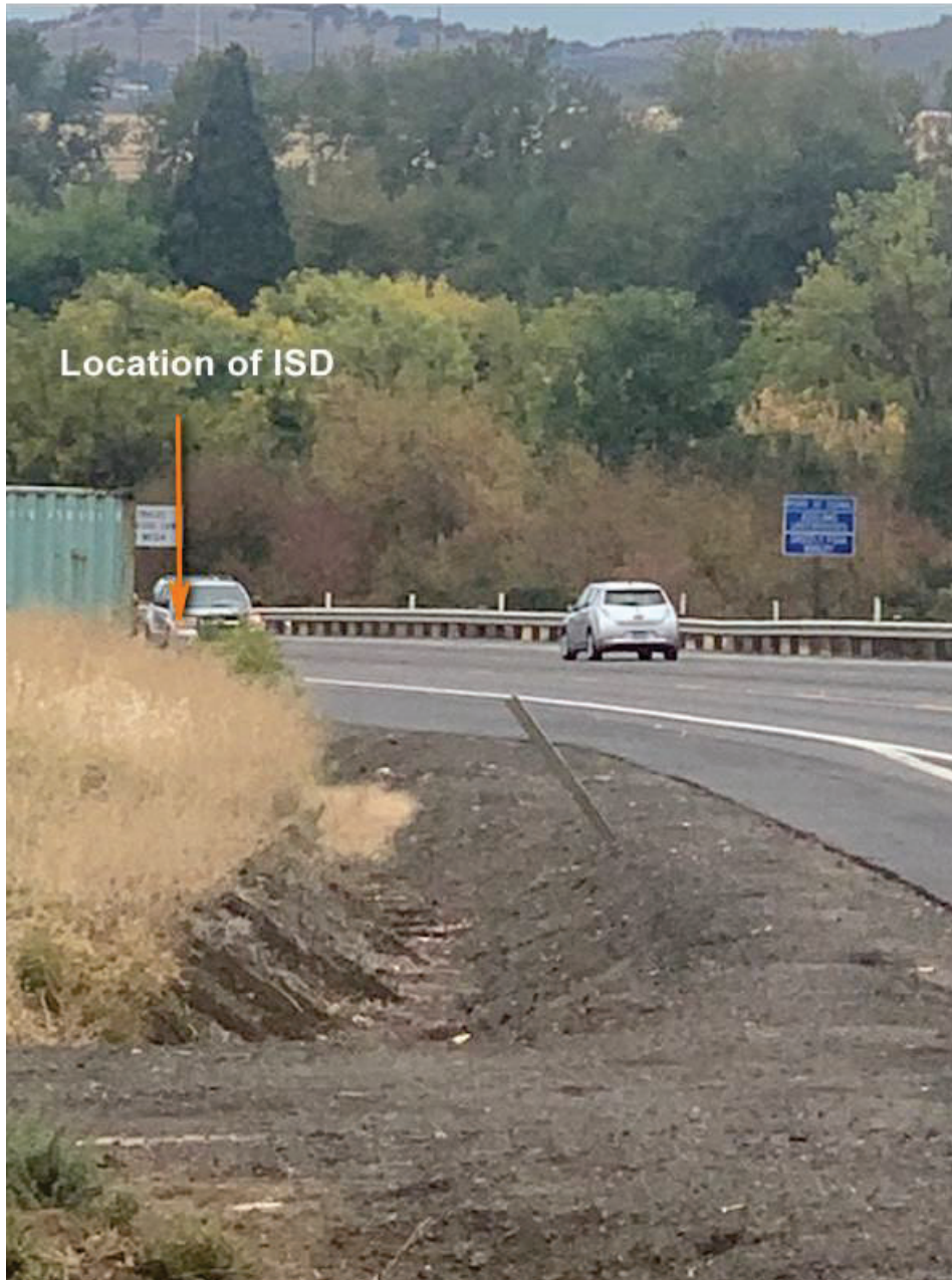
ISD requirement looking north from site access-zoomed in. ISD is met
