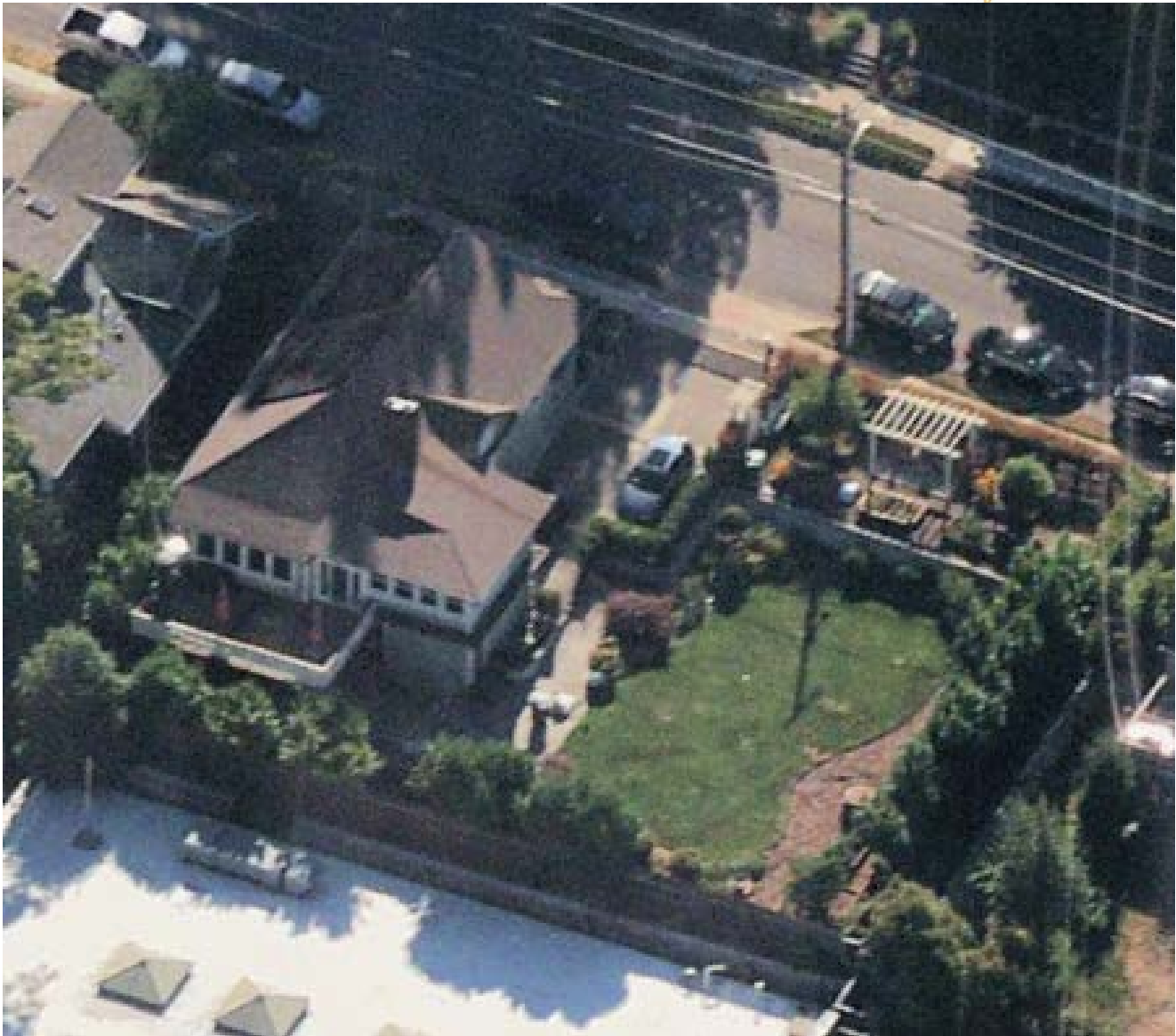
52 Granite Street (rear). Rear deck (Nearmap Image).
