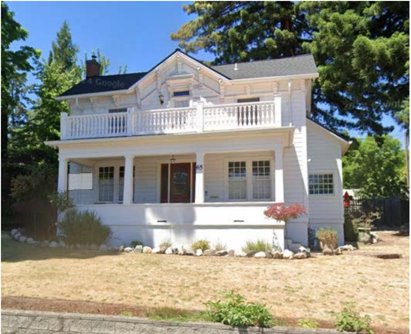
65 Granite Street. Front porch and second-story deck (Google Streetview).
