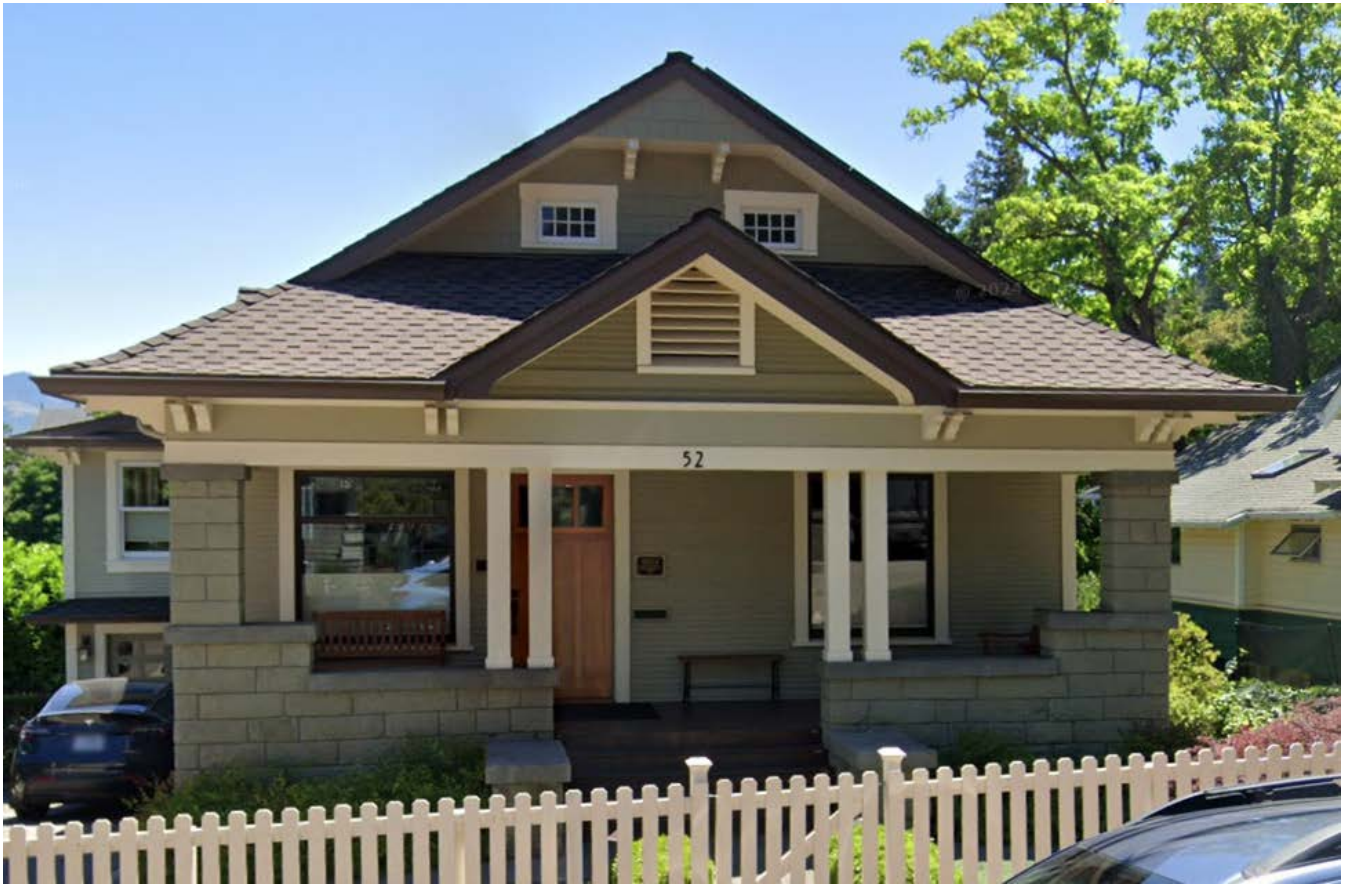
52 Granite Street (front). Original front porch (Google Streetview).
