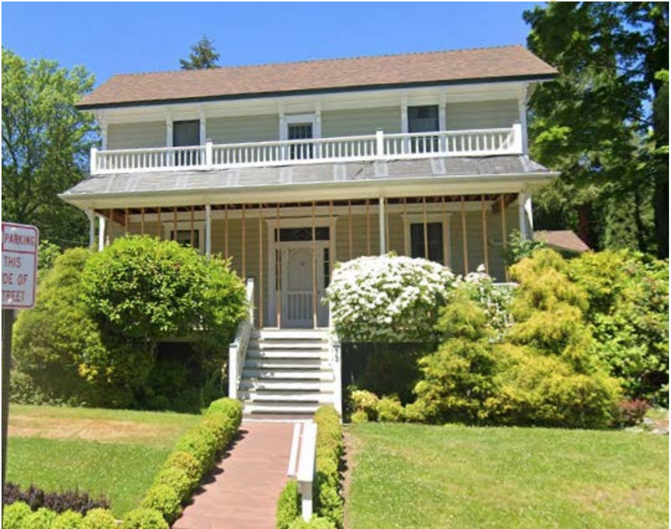
73 Granite Street. Front porch and second-story deck, rehabilitation underway (Google Streetview).
