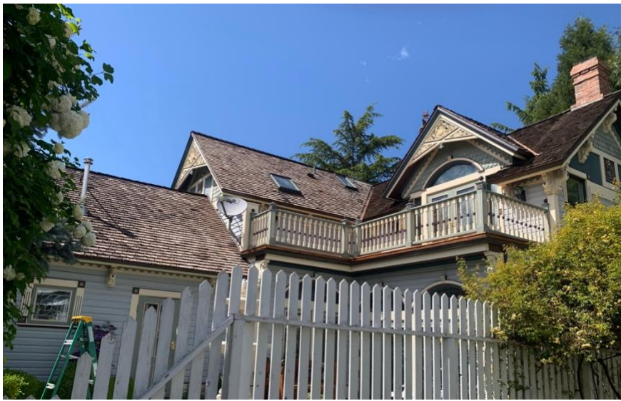
Figure 31: Wood Shake Roof, Photo Courtesy of Charisse Sydoriak
