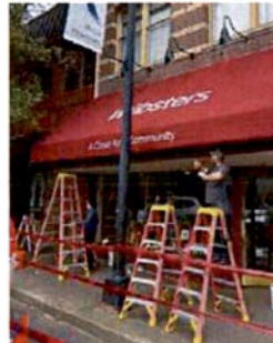
A new awning at Websters.
