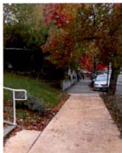
Repaired sidewalks at 450 Siskiyou.
