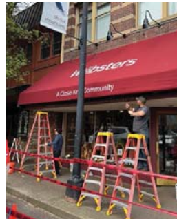
A new awning at Websters.
