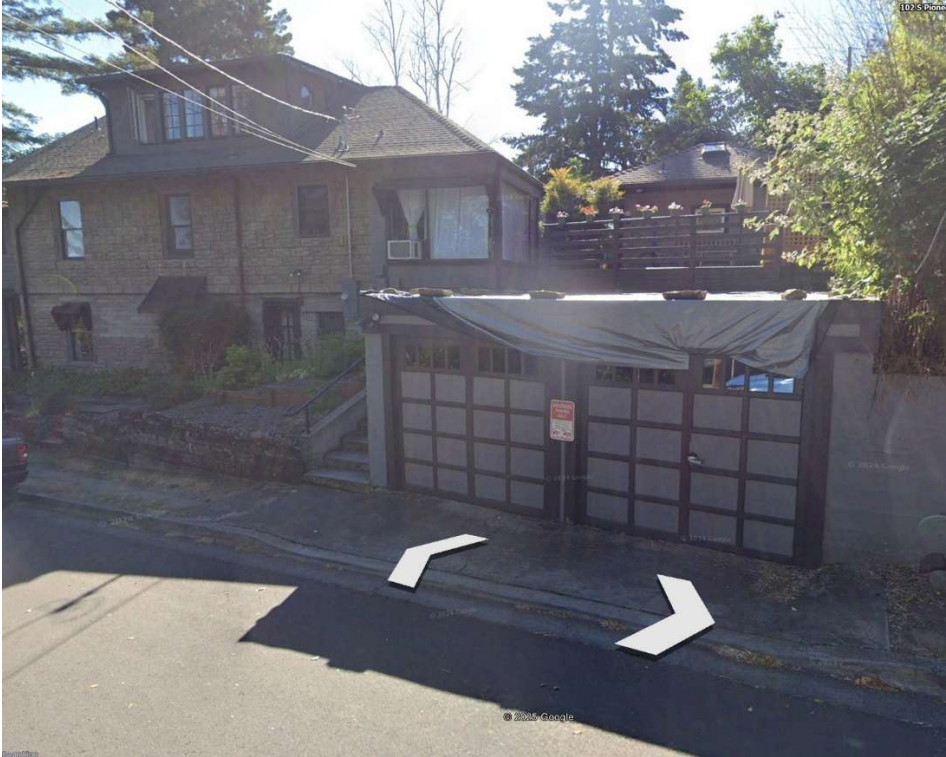
Figure 4 – Existing Garage, Residence and Studio beyond (looking East from Pioneer St.).
