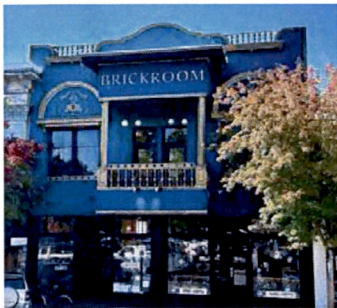
Fresh coat of paint, signage and lighting at the Brickroom.
