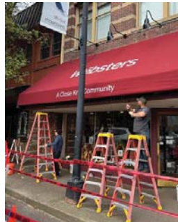
A new awning at Websters.
