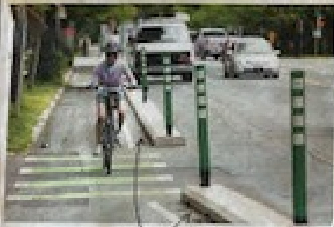
Concrete curbing WITH posts
