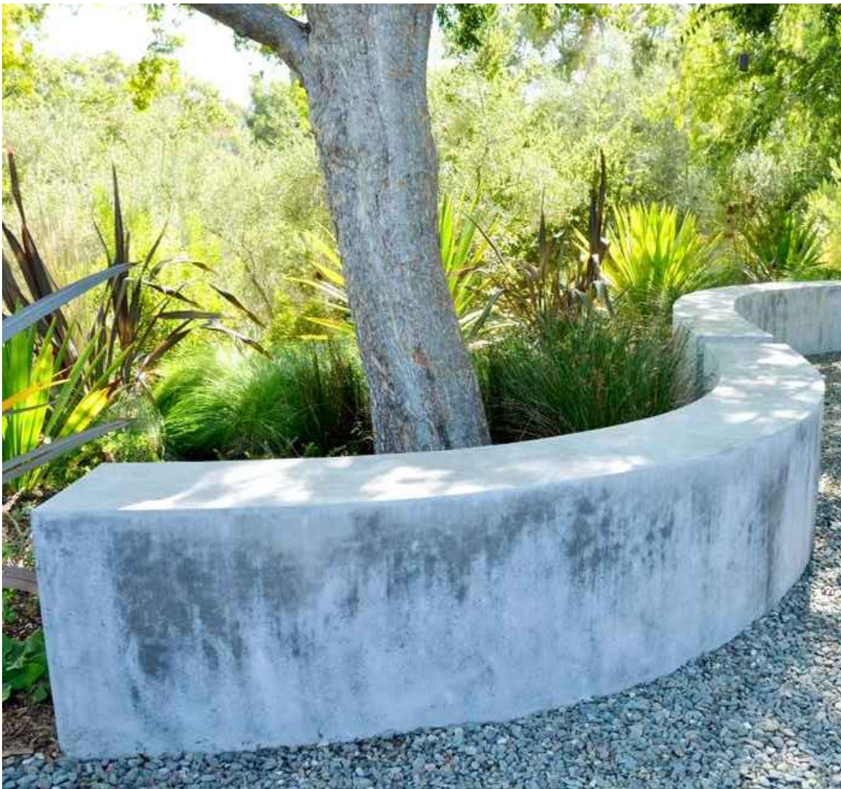
6 PRECEDENT IMAGE: 24" MAX CONCRETE SEATWALL Scale: NTS
