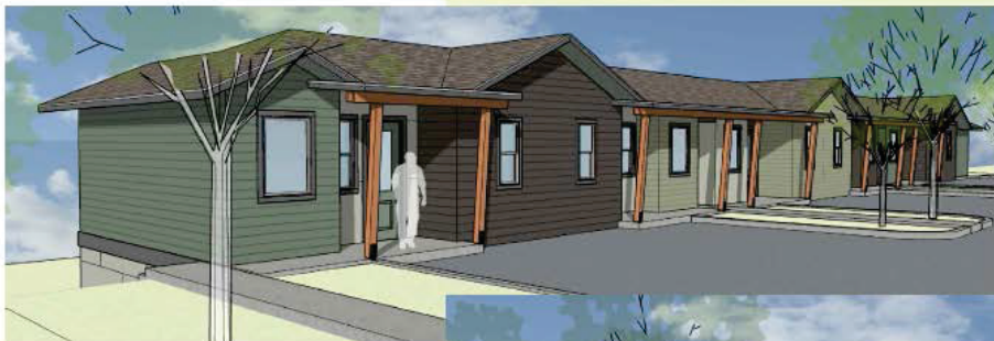
MARIPOSA COURT VIEW
